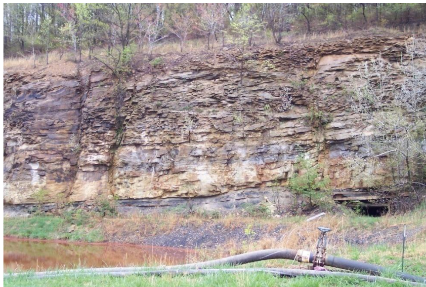
Figure 2-6. Omega Mine Face-up Area Showing Vertical Fractures in Sandstone Overburden. Partially Open Mine Entry at Right.
